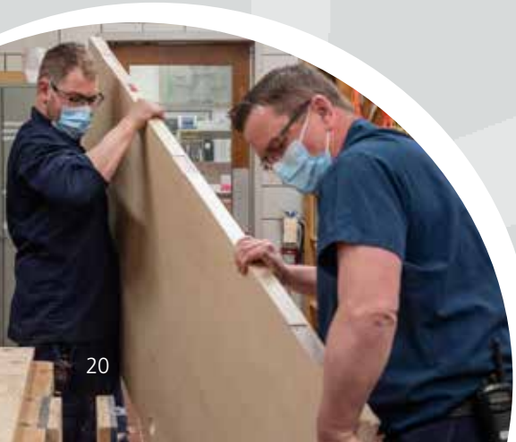
Maintenance staff Joel Kreuger and Werner Spenst repairing a door.
